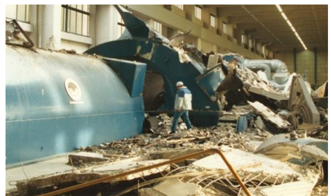
Fig. 9: Catastrophic failure of steam turbine caused by a sudden rupture of the turbine shaft
