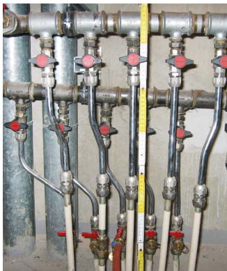
Typical water pipe arrangement in buildings
