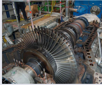
Steam turbine opened for maintenance
